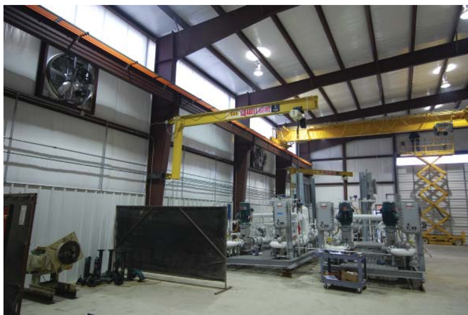
The project adds another 7,000 sq ft to Chemtec's existing shop space
