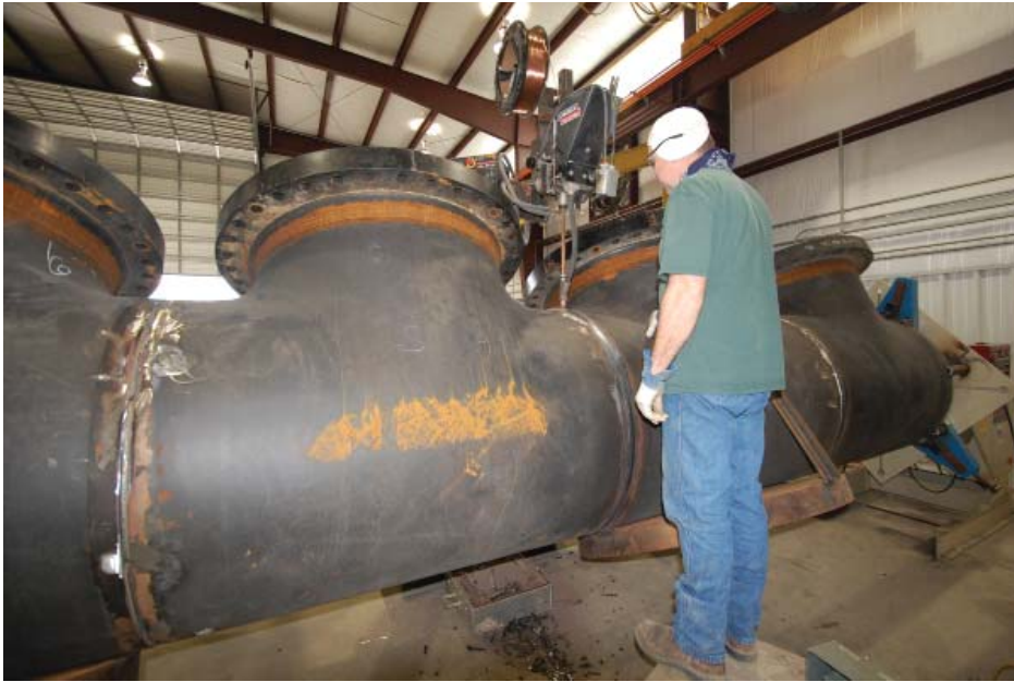
Chemtec has been fabricating large-bore pipe spools for Magellan Midstream Partners
